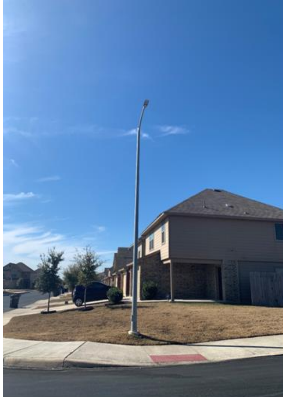
Existing CPS Energy Pole
