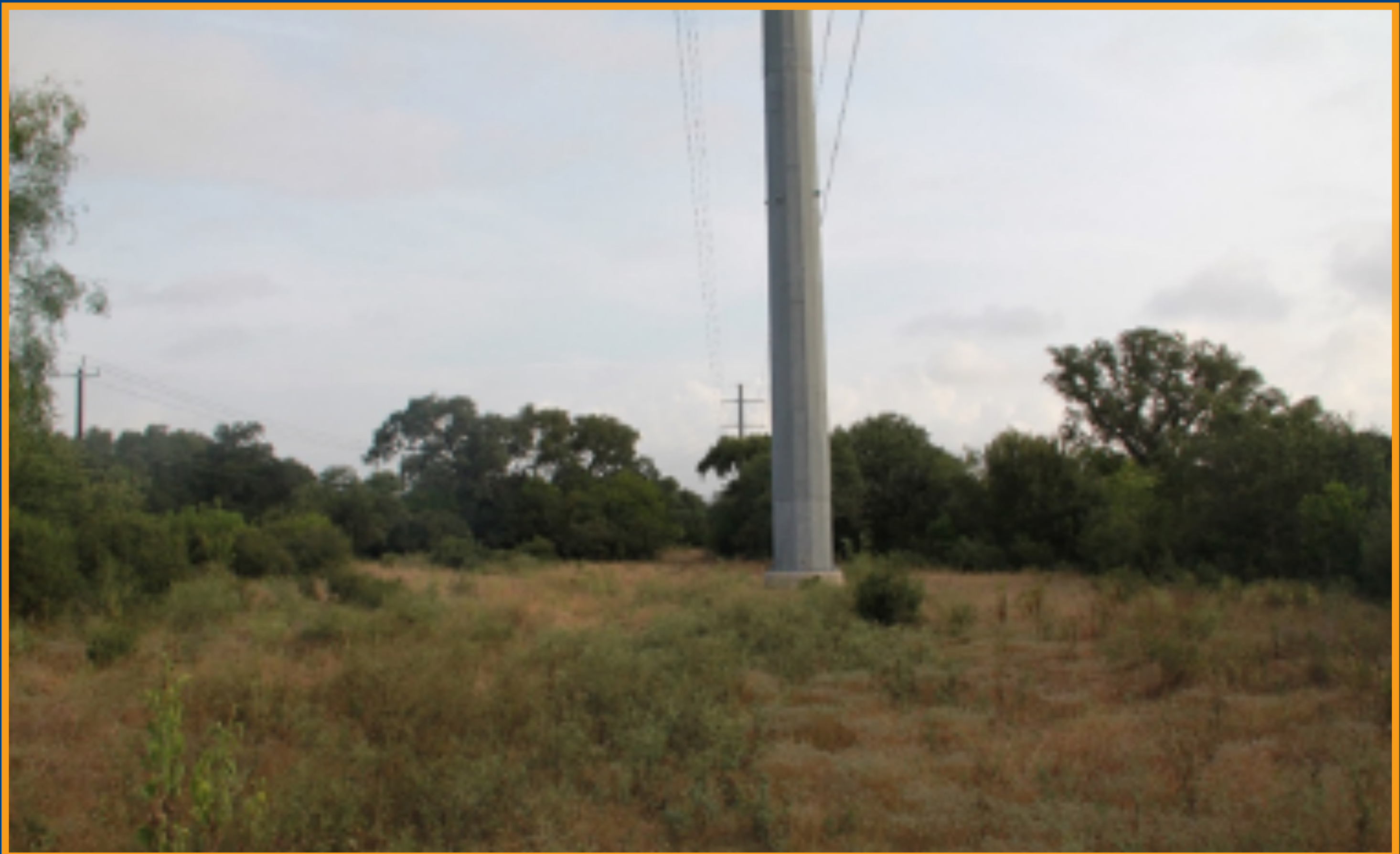
Clearing around transmission poles
