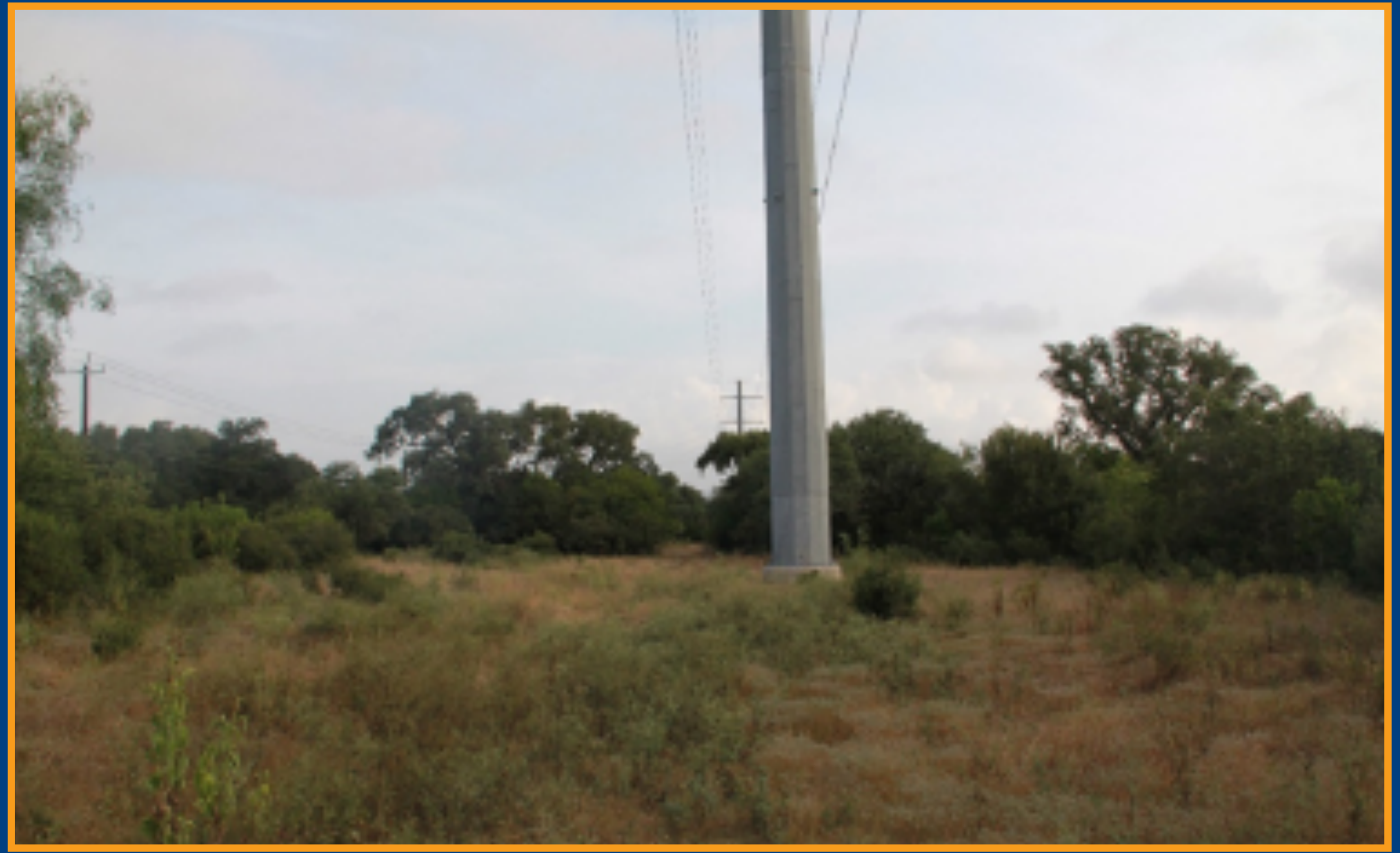
Clearing around transmission poles
