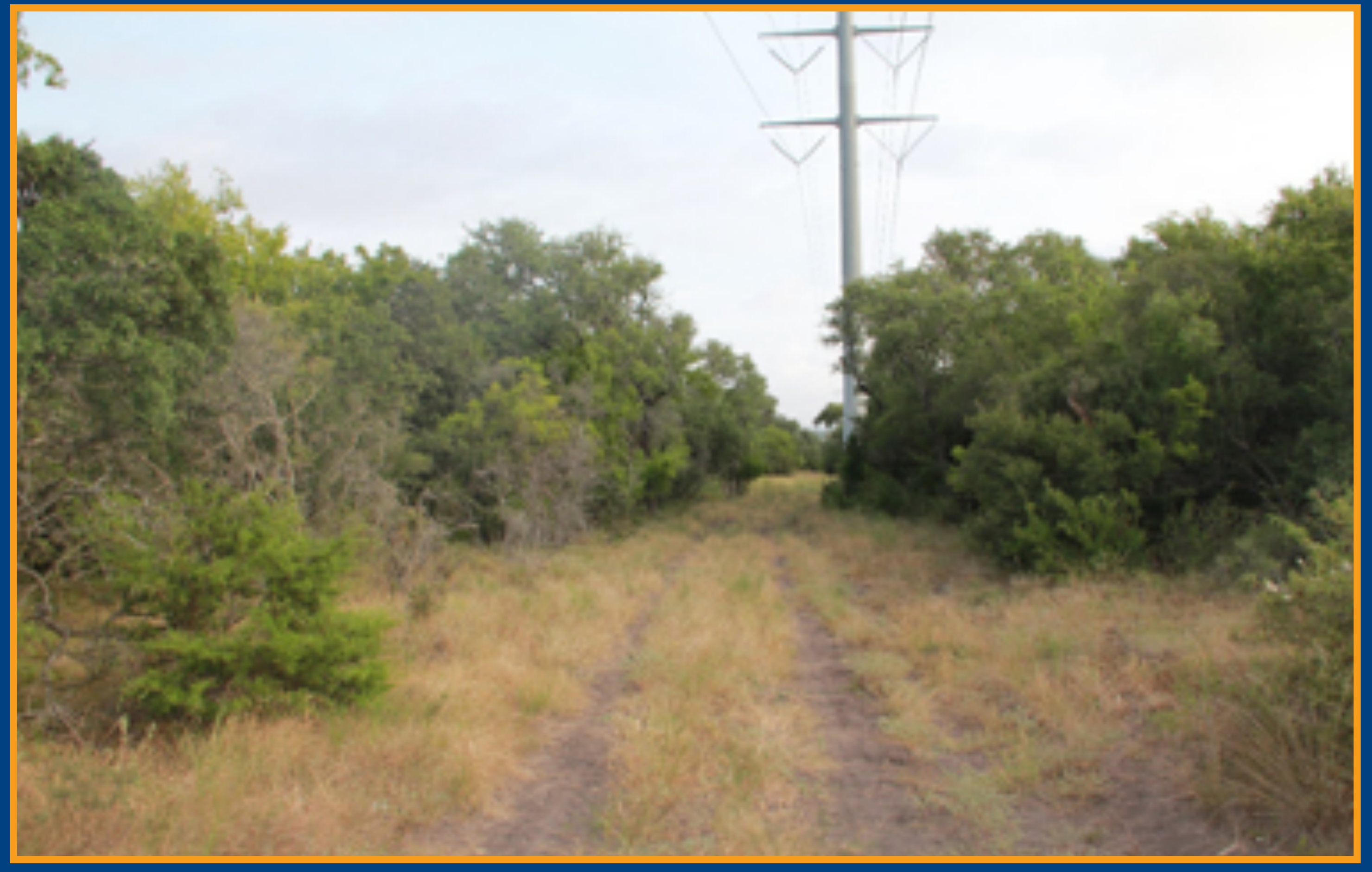
Clearing along route
