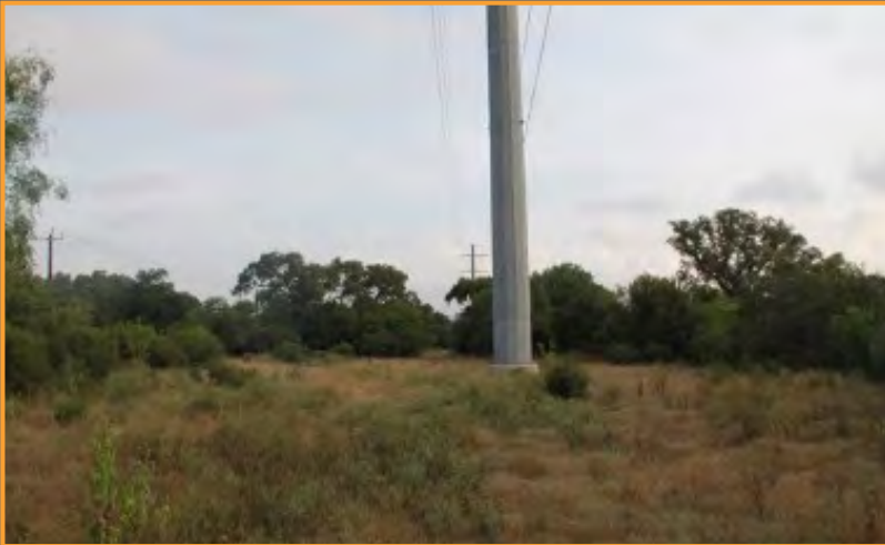
Clearing around transmission poles
