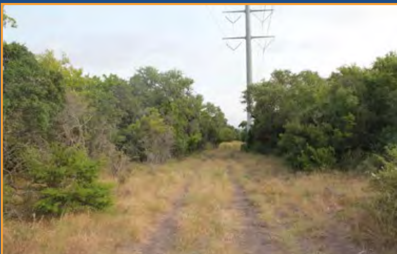
Clearing along route
