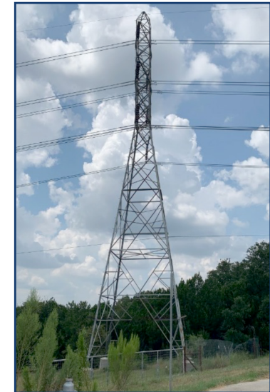
Existing Lattice Structure
