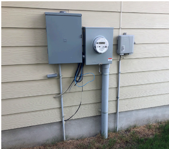
Typical Underground Meter Loop
