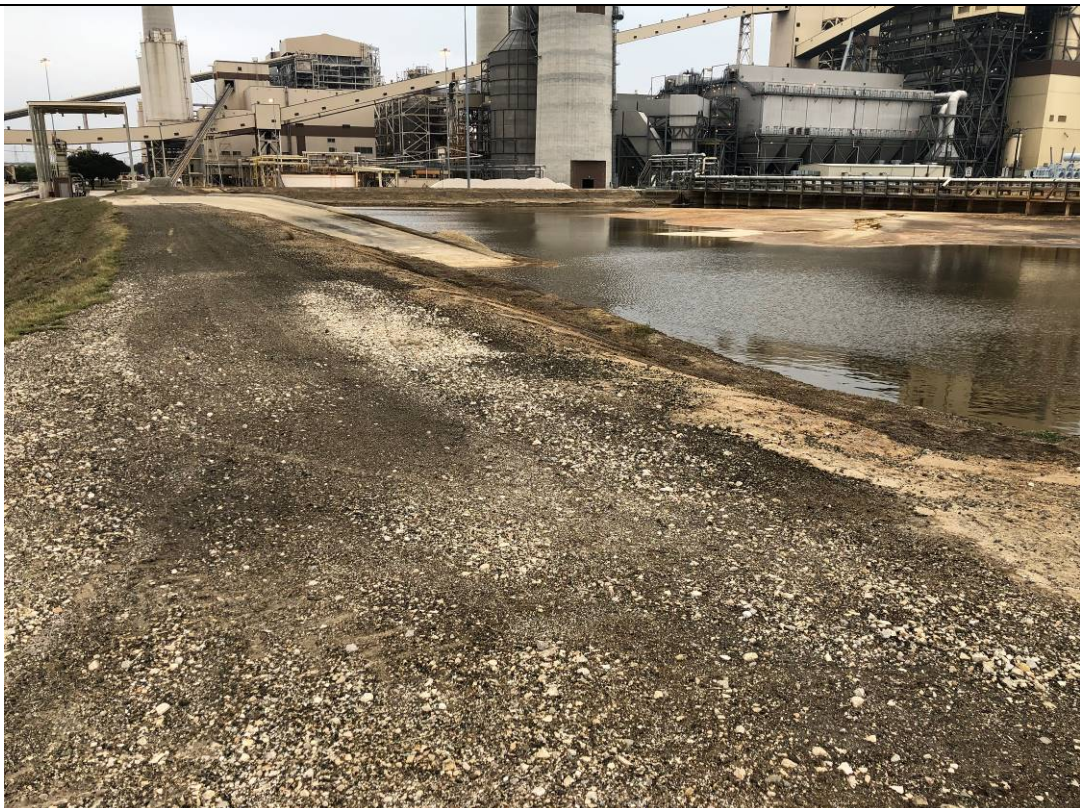
Photograph: 34 South SRH Pond – standing on the southeast corner – facing west. Photo taken 12/15/2020.
