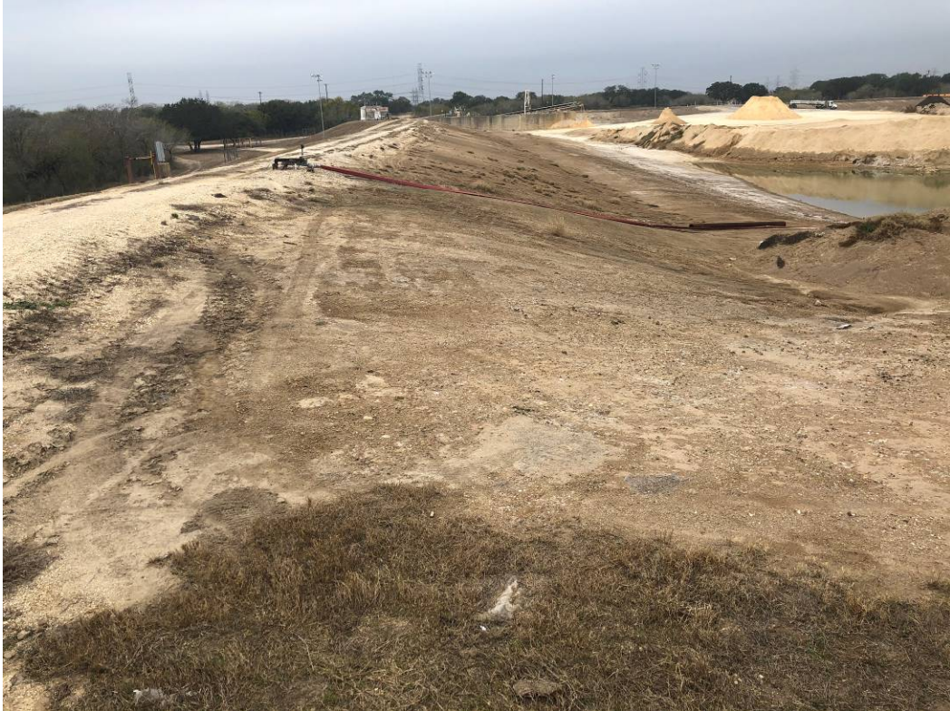
Photograph: 5 Fly Ash Landfill – standing on southeast corner – facing west. Radial stacker located in southwest corner and stormwater discharge piping in southeast corner of landfill. Photo taken 12/15/2020.
