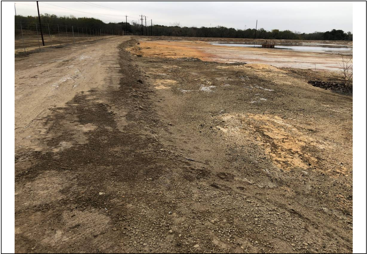
Photograph: 11 | Evaporation Pond – standing on the southwest corner – facing north. Photo taken 12/15/2020.
