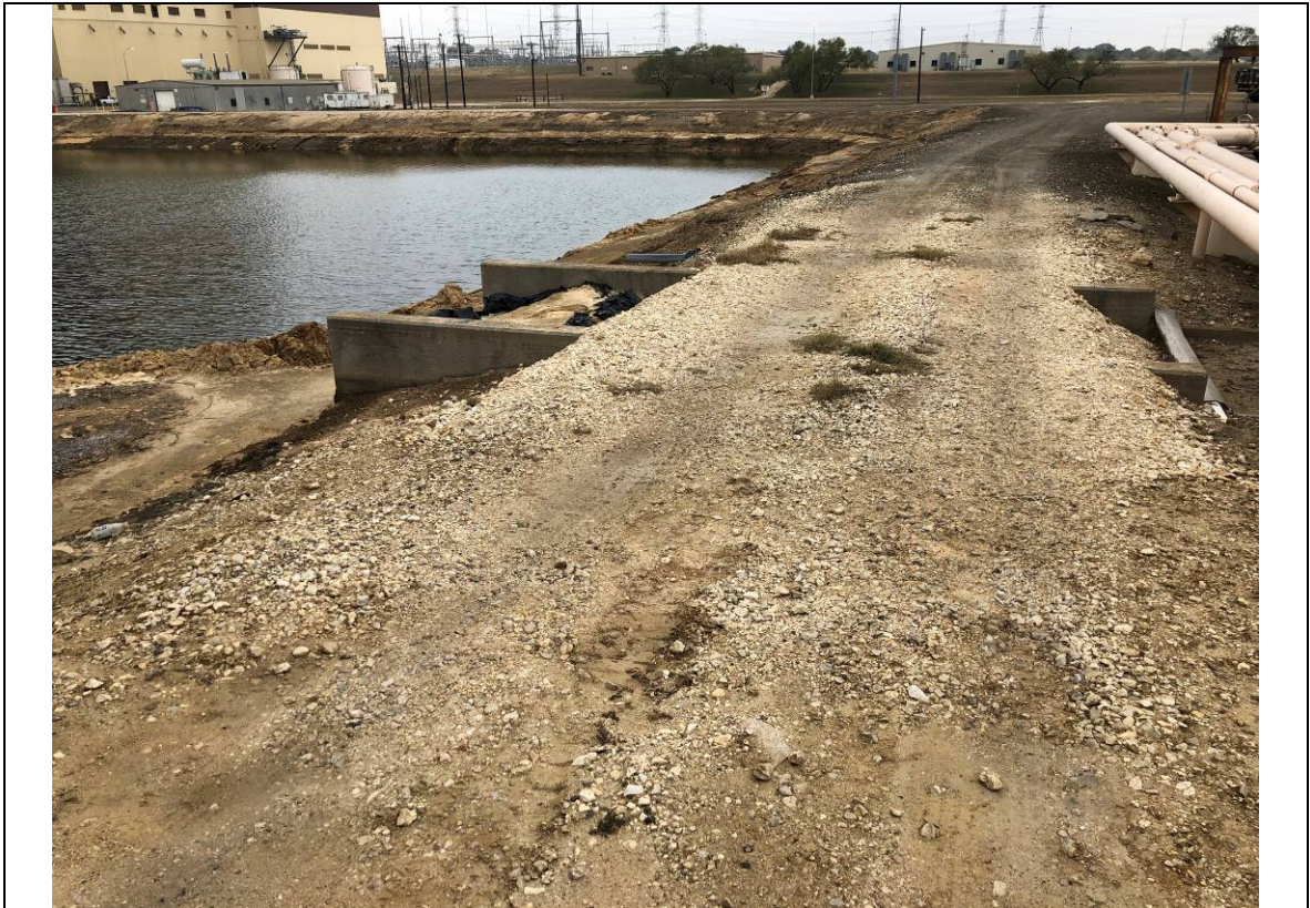
Photograph: 29 North SRH Pond – standing on southeast corner – facing north. Spillway structure. Photo taken 12/15/2020.
