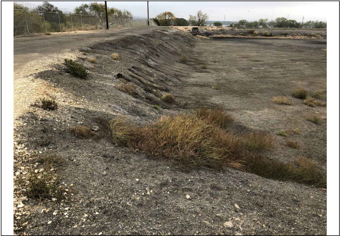
Photograph: 17 North Bottom Ash Pond – standing on northwest corner – facing east. Photo taken 12/15/2020.
