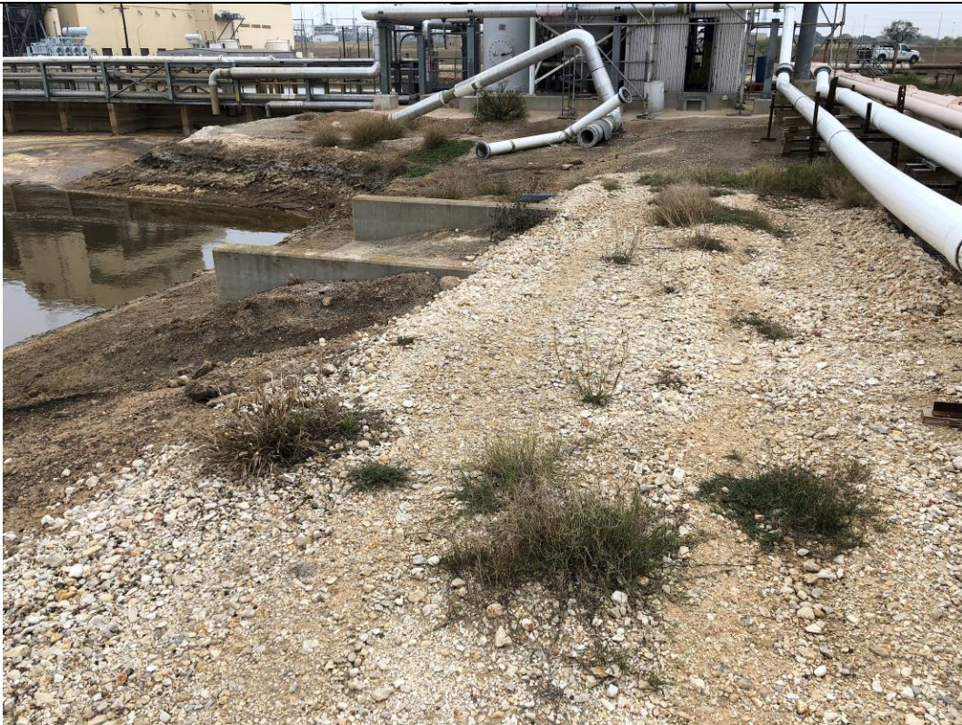
Photograph: 36 South SRH Pond – standing on east corner – facing north. Spillway structure. Photo taken 12/15/2020.
