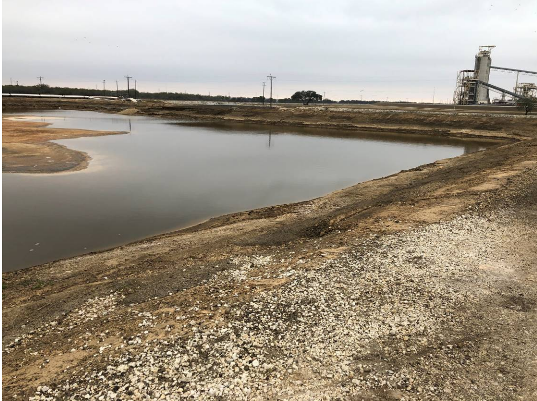
Photograph: 31 | South SRH Pond – standing on the northwest corner – facing southeast. Photo taken 12/15/2020.
