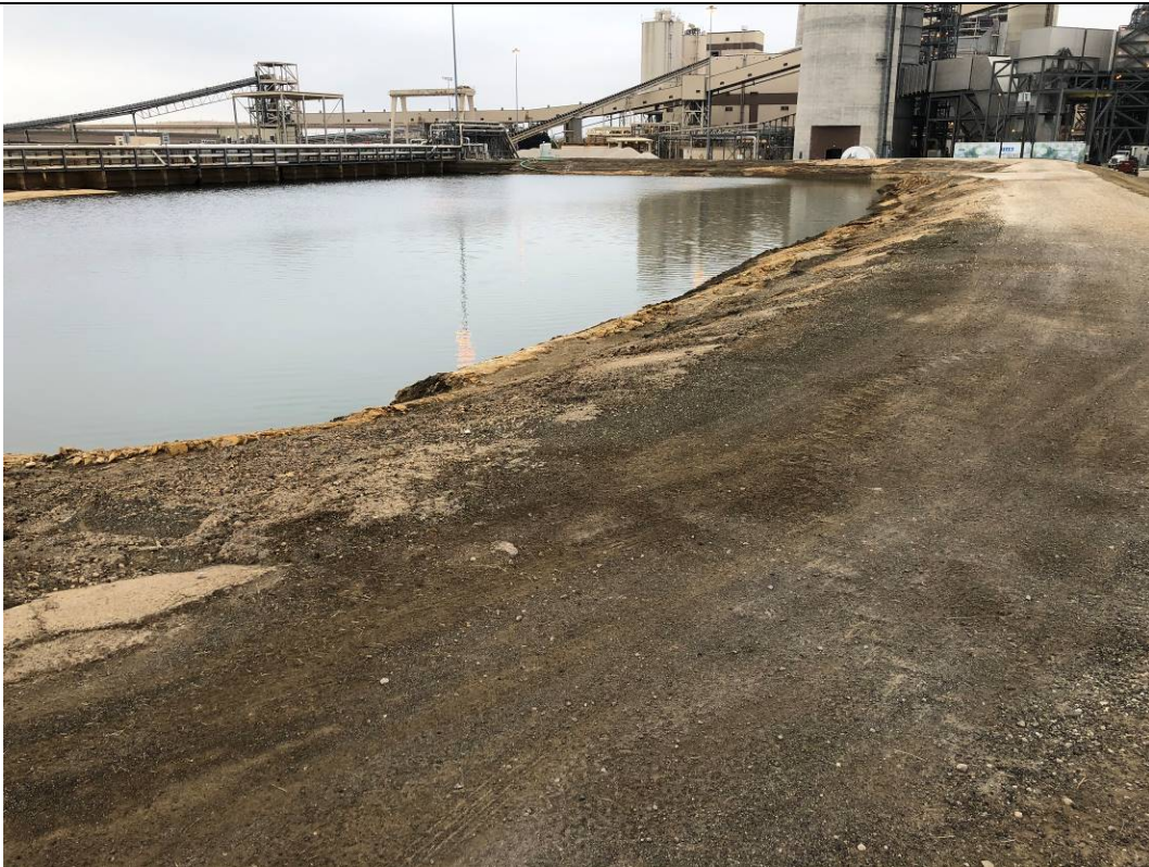
Photograph: 26 North SRH Pond – standing on northeast corner – facing west. Photo taken 12/15/2020.
