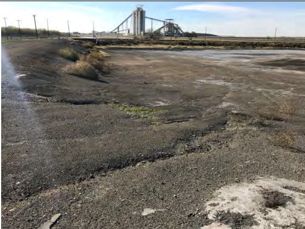
Photograph: 20 South Bottom Ash Pond – standing on northeast corner – facing south. Photo taken 12/19/2019.
