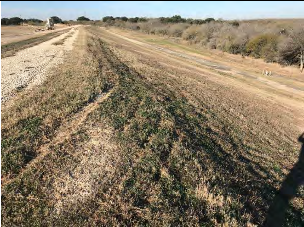
Photograph: 2 Fly Ash Landfill – standing on northern berm – facing west. Photo taken 12/19/2019.
