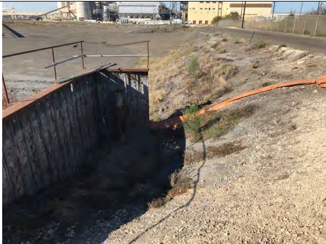
Photograph: 16 North Bottom Ash Pond – standing on northwest corner – facing east. Photo taken 12/19/2019. Corrosion observed in vertical overflow pipe and sheet piling.
