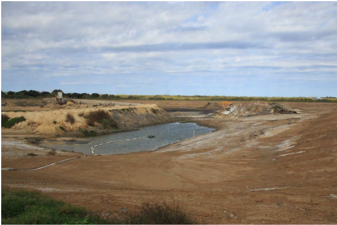
Photograph: 5 Fly Ash Landfill – standing on southeast corner of landfill – facing north. Rain water accumulates in southeast corner of landfill. Photo taken 12/16/15.
