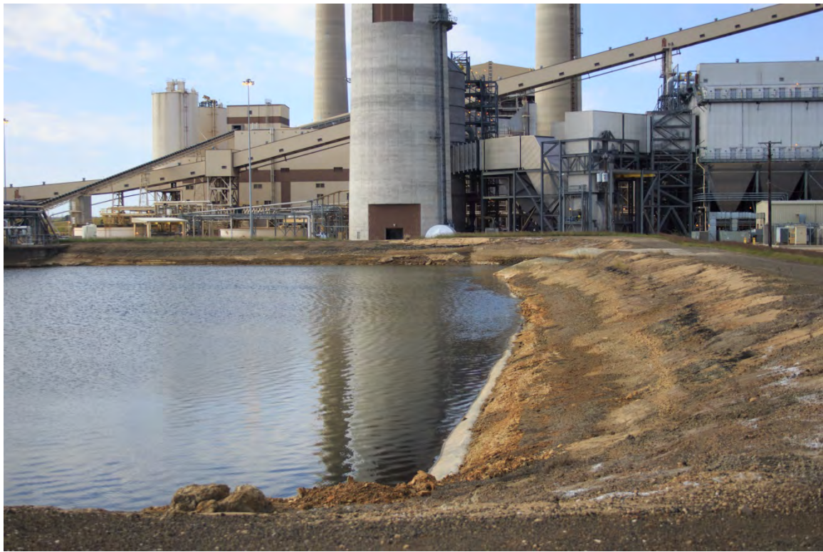
Photograph: 17 North SRH Pond – standing on northeast corner of pond – facing west. Photo taken 12/16/15.
