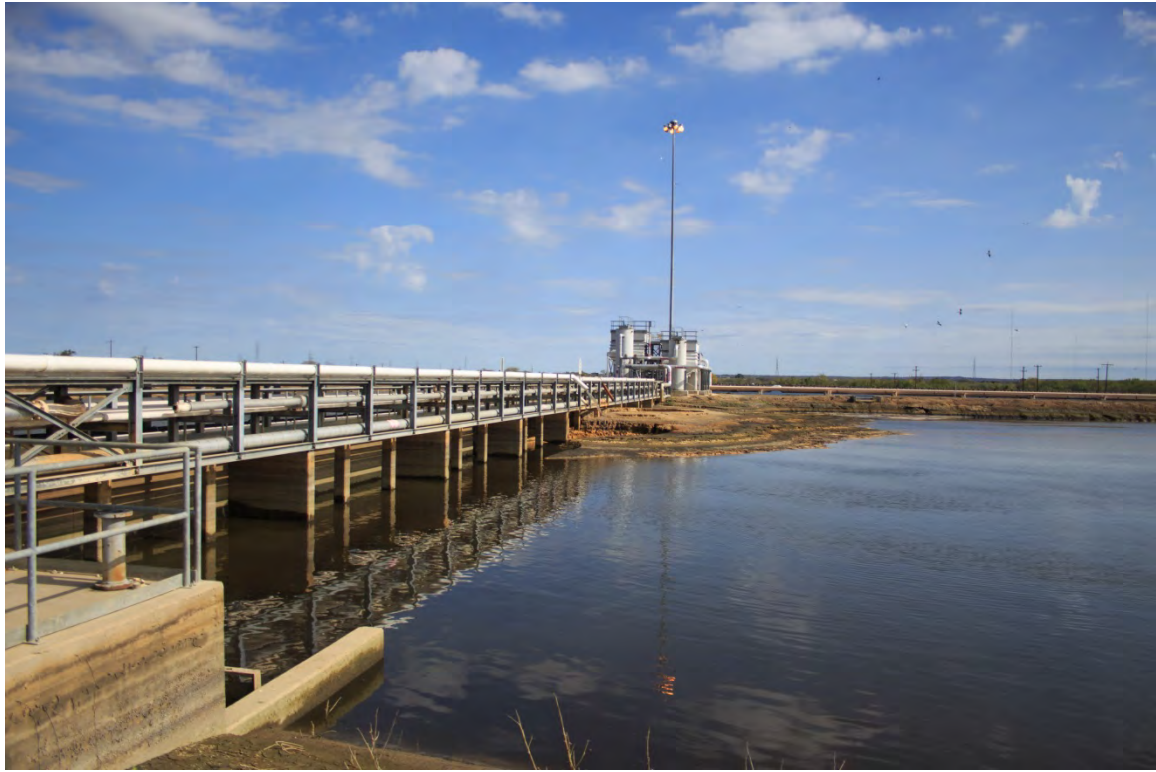
Photograph: 21 South SRH Pond – standing on western berm – facing east. Photo taken 12/16/15.
