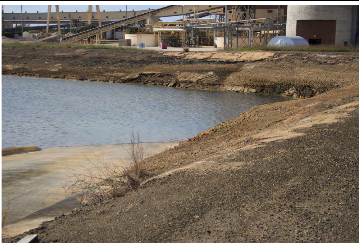
Photograph: 20 North SRH Pond – standing on northern berm – facing southwest. Erosional features on western berm. Photo taken 12/16/15.
