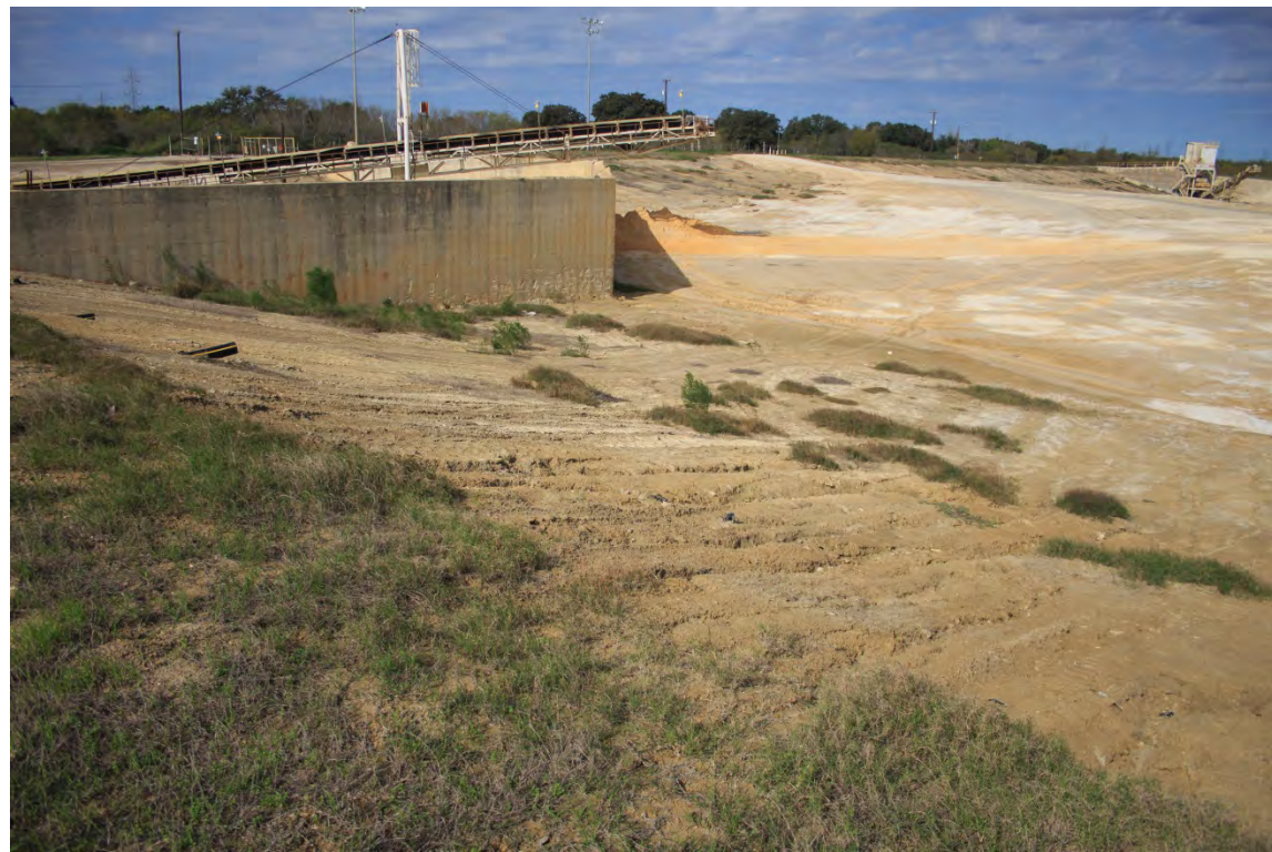
Photograph: 6 Fly Ash Landfill – standing on southern berm – facing northwest. Erosion features on southern berm near radial stacker. Photo taken 12/16/15.
