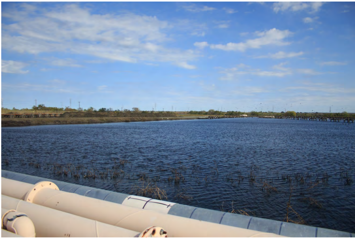
Photograph: 25 South Bottom Ash Pond – standing on western berm – facing northeast. Photo taken 12/16/15.
