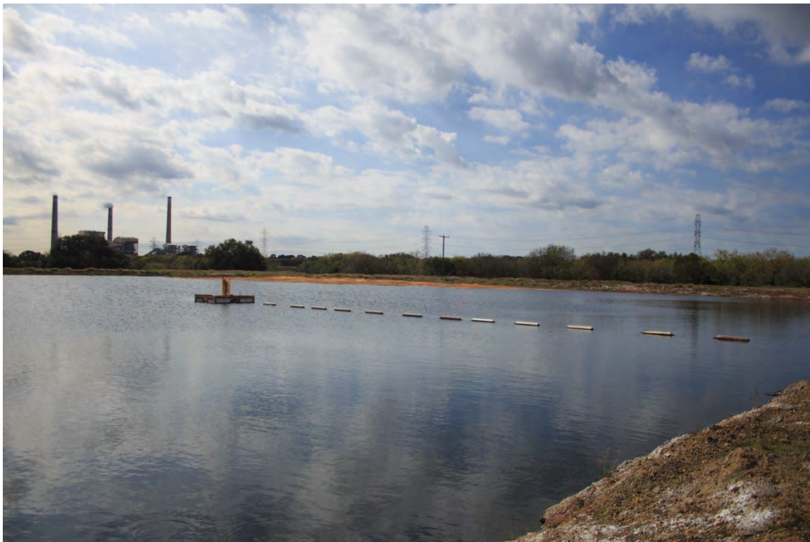
Photograph: 9 Evaporation Pond – standing on northern berm – facing southwest. Photo taken 12/16/15.
