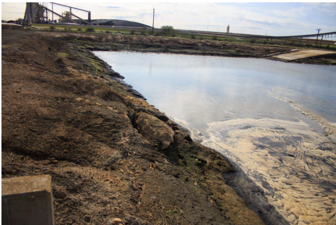
Photograph: 24 South SRH Pond – standing on eastern berm – facing south. Erosional features on eastern berm. Photo taken 12/16/15.
