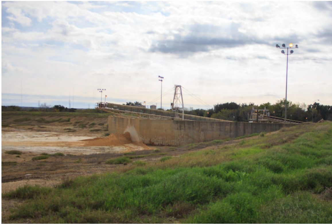
Photograph: 3 Fly Ash Landfill – standing on western berm – facing southeast. Radial stacker located in southwest corner of landfill. Photo taken 12/16/15.
