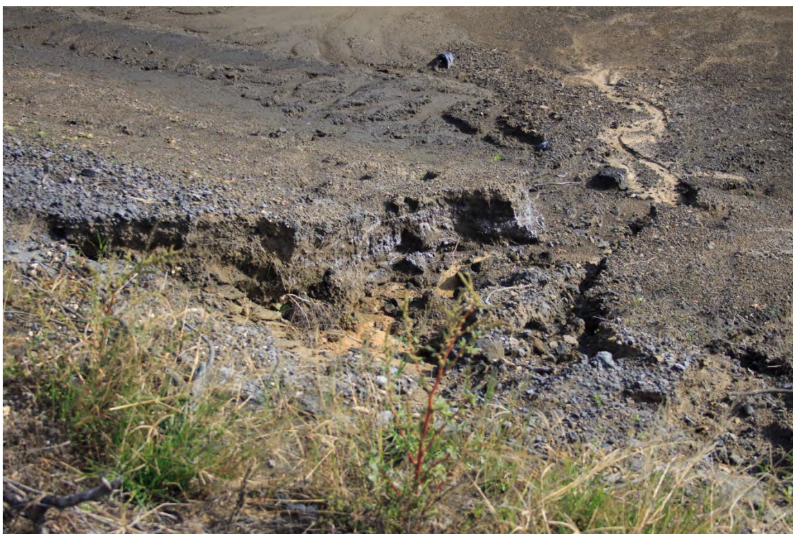
Photograph: 14 North Bottom Ash Pond – standing on western berm – facing east. Erosion features on inside of western berm. Photo taken 12/16/15.
