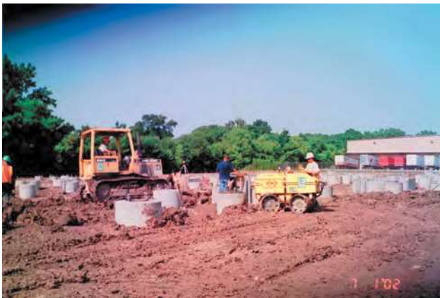
Figure 5-4 Placement and compaction of compacted clay around existing structures
