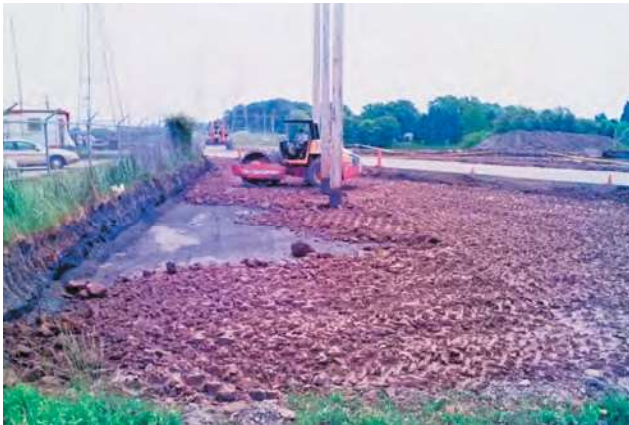
Figure 5-3 Placement and compaction of a clay barrier in a cap application using a sheepsfoot roller
