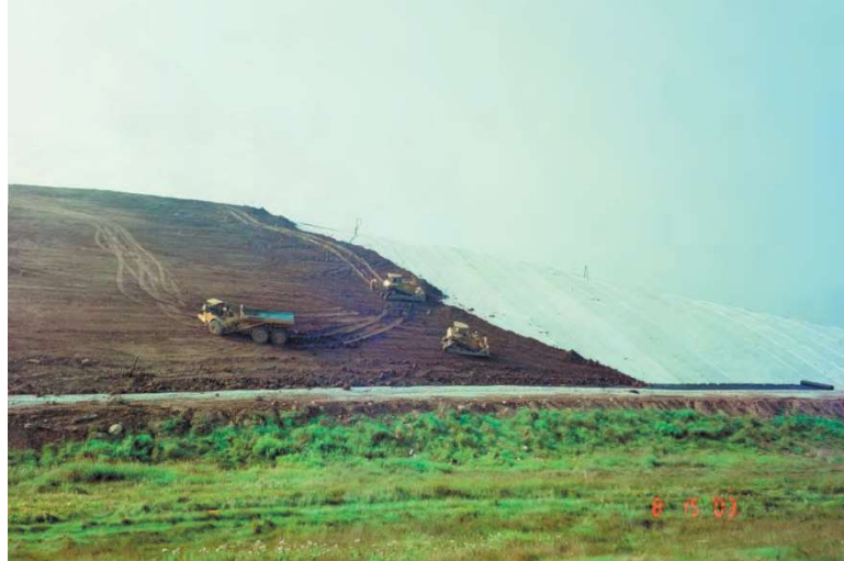
Figure 5-1 Placement of a cover layer
