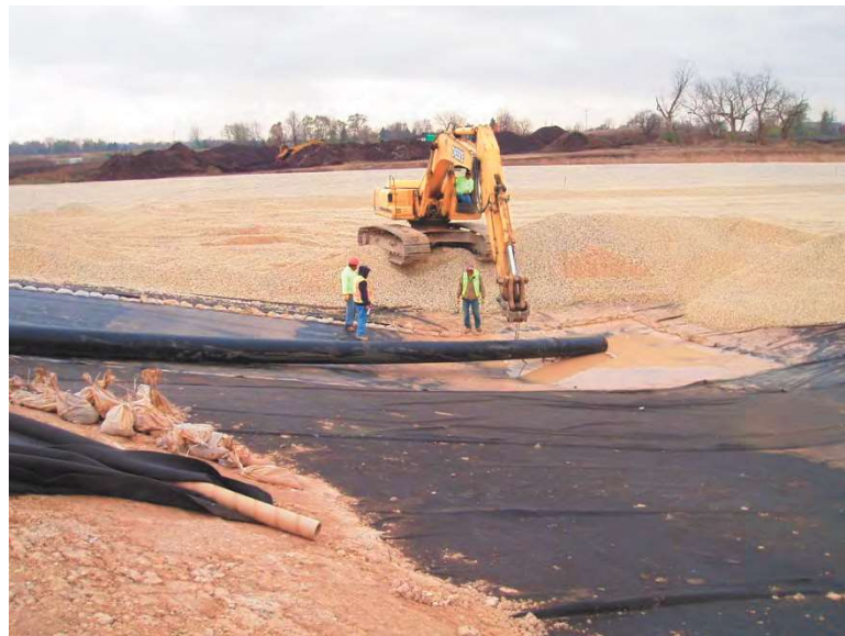
Figure 4-6 Sideslope riser pipe being installed in a leachate collection sump
