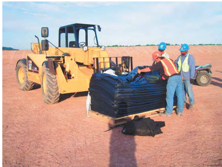
Figure 3-8 Geomembrane accordion folded on a pallet prior to deployment
