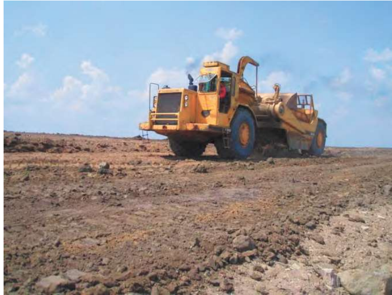
Figure 3-2 Grading a compacted clay liner
