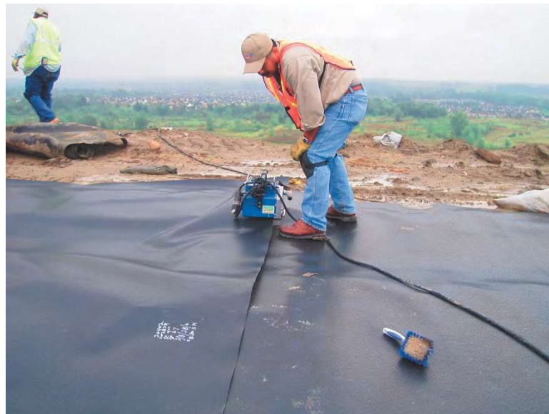
Figure 3-3 Thermal fusion welding HDPE geomembrane sheets together in the field
