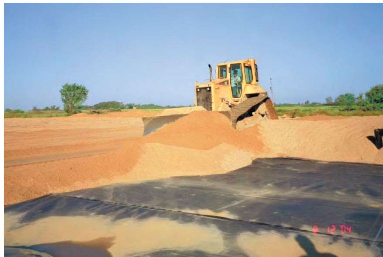
Figure 4-2 Granular drainage blanket placement over a 60-mil HDPE Geomembrane
