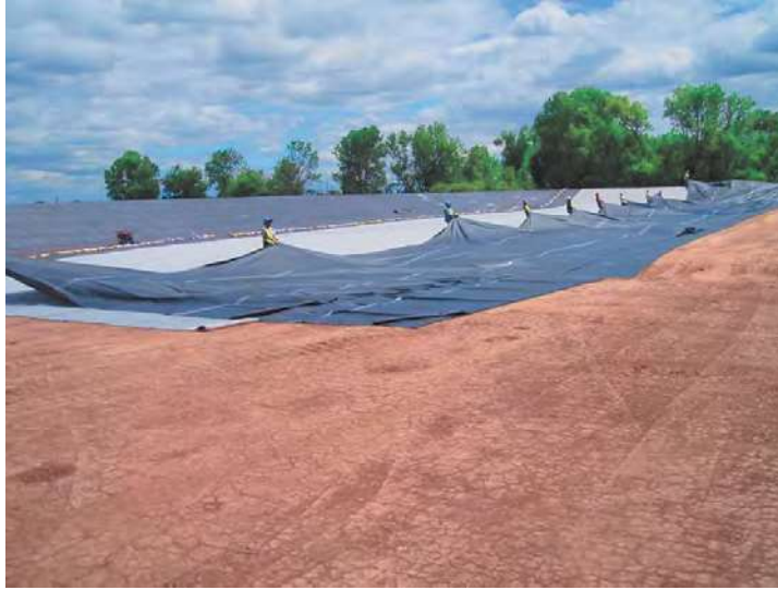
Figure 3-9 Deployment of a large factory fabricated sheet of PVC geomembrane
