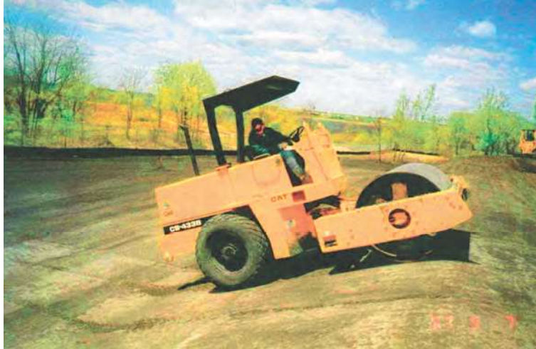
Figure 5-13 Compaction operations for a cap incorporating stabilized/solidified fly ash
