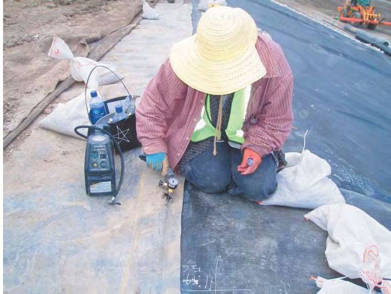
Figure 3-4 Nondestructive pressure testing of a dual-track fusion weld
