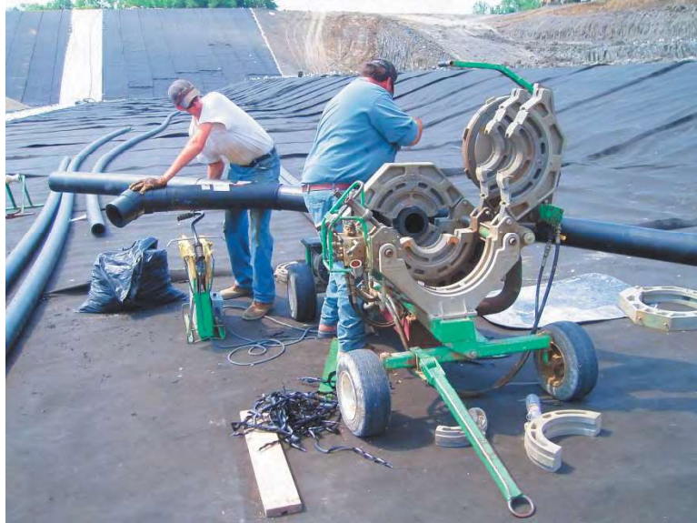
Figure 4-4 Assembly of HDPE leachate collection pipe by means of fusion welding
