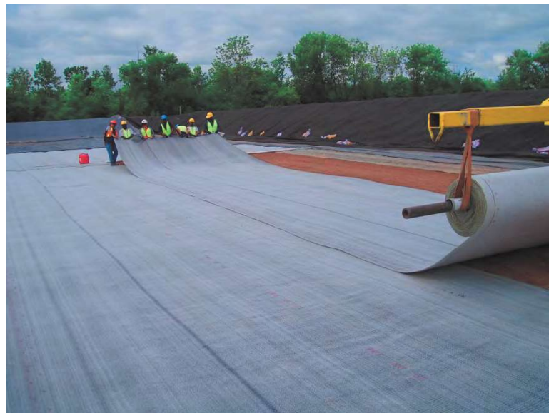
Figure 3-13 Typical GCL installation, showing removal from the roll and overlapping panels
