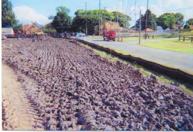
Figure 5-3 Placement and compaction of a clay barrier in a cap application using a sheepsfoot roller
