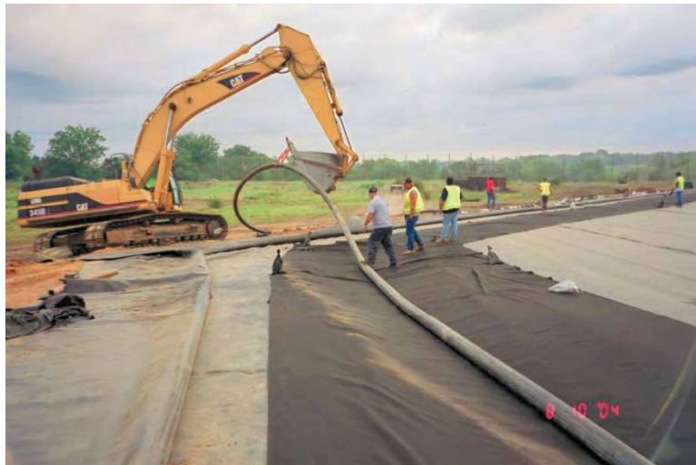
Figure 4-5 Installation of leachate collection pipe in the leachate collection trench
