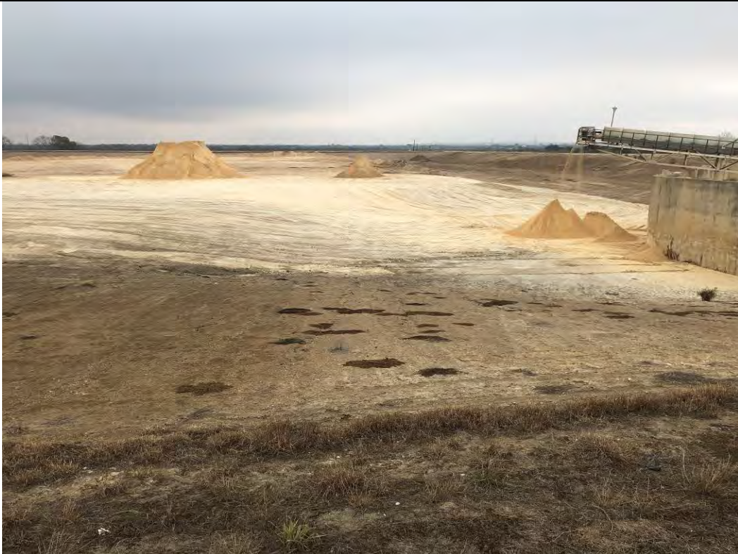
Photograph: 1 Fly Ash Landfill – standing on west berm – facing east. Radial stacker located in southwest corner of landfill. Photo taken 12/15/2020.
