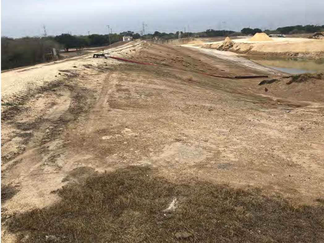
Photograph: 5 Fly Ash Landfill – standing on southeast corner – facing west. Radial stacker located in southwest corner and stormwater discharge piping in southeast corner of landfill. Photo taken 12/15/2020.
