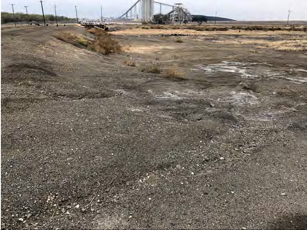
Photograph: 21 South Bottom Ash Pond – standing on northeast corner – facing south. Photo taken 12/15/2020.
