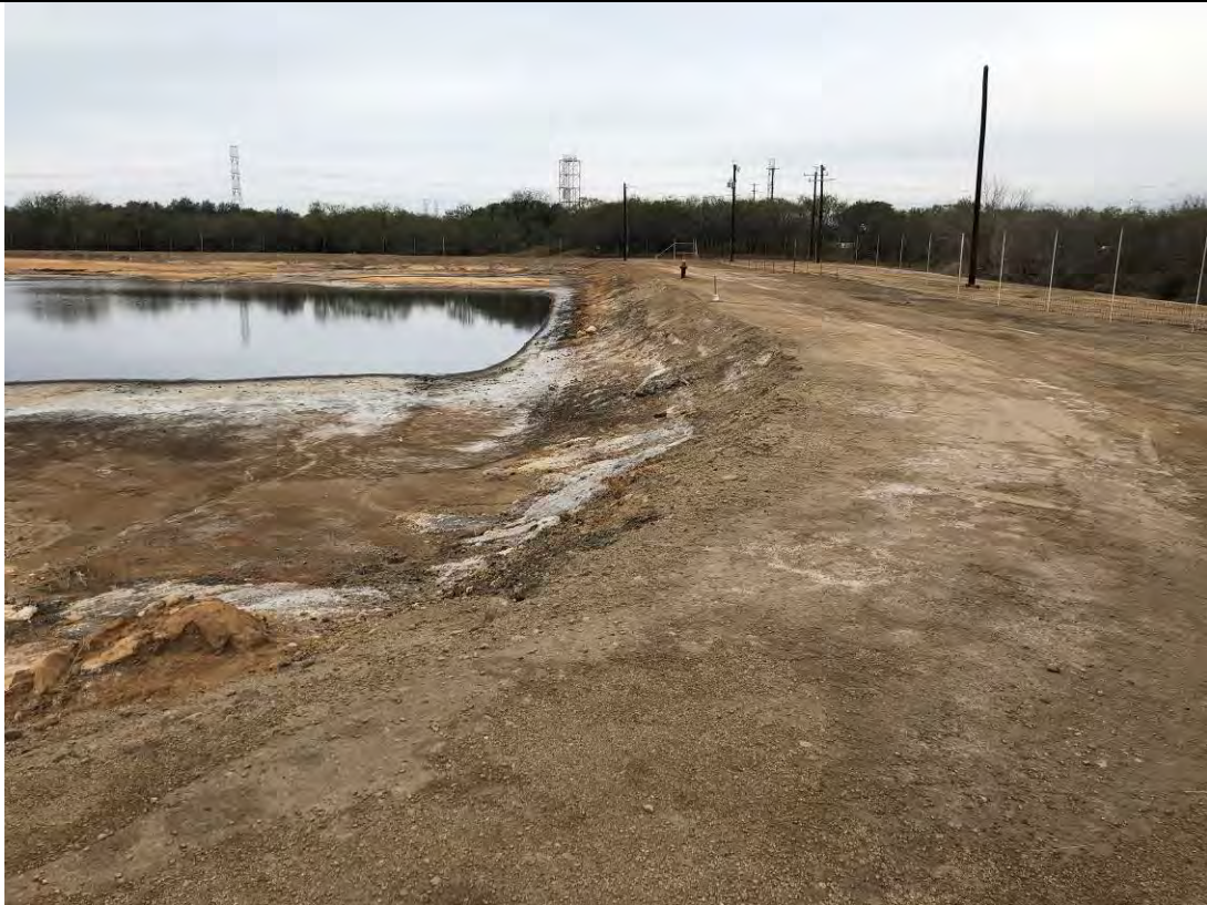
Photograph: 9 Evaporation Pond – standing on the northeast corner – facing west. Photo taken 12/15/2020.
