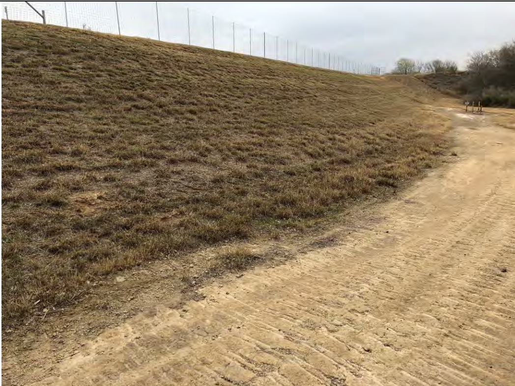
Photograph: 16 Evaporation Pond – standing on the southwest corner – facing east. Photo taken 12/15/2020.
